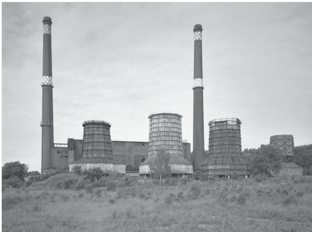
Plessa power station Elektrárň v Plessa
