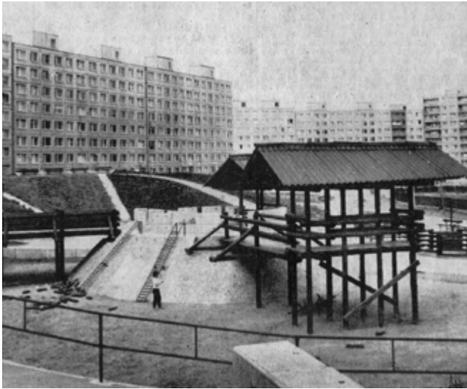
LANDSCAPING OF A BLOCK, SOUTHWEST CITY HOUSING ESTATE IN PRAGUE, IVO OBERSTEIN, MILAN KLÍMA, IVAN HOŘEJŠÍ, MARTIN KOTÍK, VÁCLAV VALTR, EVŽEN STEIN, ETC., 1967–1991
