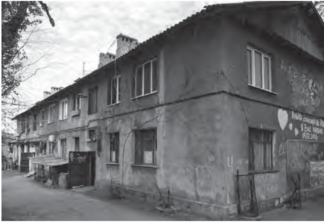
ODESSA, RESIDENTIAL HOUSE OF GYPSUM CANE-FIBRE BOARD, DESIGNED FOR 16 APARTMENTS (1 – 2 ROOMS). OBLPROEKT DESIGN ORGANIZATION. ENG. RENDINO S., GOLDBERG D., 1960
