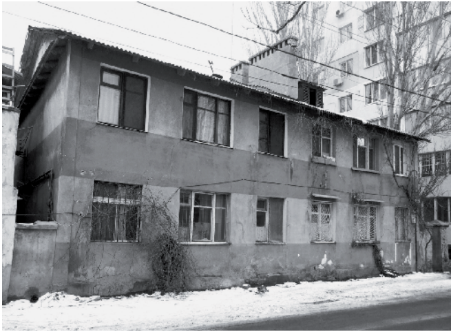
ODESSA, RESIDENTIAL HOUSE OF GYPSUM CANE-FIBRE BOARD, DESIGNED FOR 8 APARTMENTS (1 – 2 ROOMS). OBLPROEKT DESIGN ORGANIZATION. ENG. RENDINO S., GOLDBERG D., 1960
