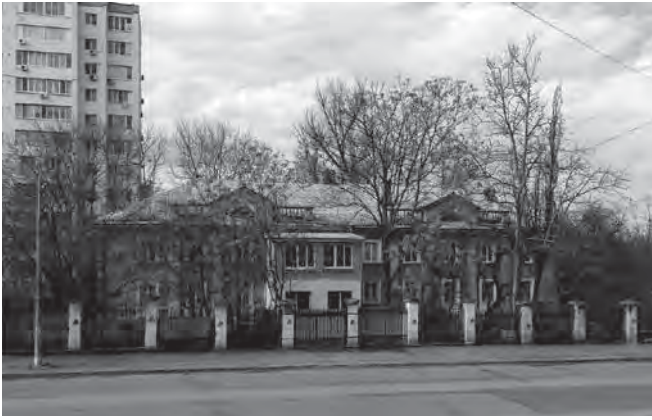
ODESSA, TWO-STOREY 16-APARTMENT RESIDENTIAL BLOCKS FOR STAFF MEMBERS OF THE INSTITUTE FOR GENETICS AND SCIENTIFIC BREEDING RESEARCH (ARCH. DRAGOMIRETSKAYA, O. T., 1950S)
