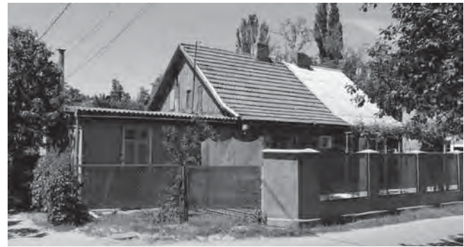
ODESSA, EXAMPLE OF POST-WAR SINGLE-STOREY HOUSE FOR TWO FAMILIES. THE LATE 1940S
