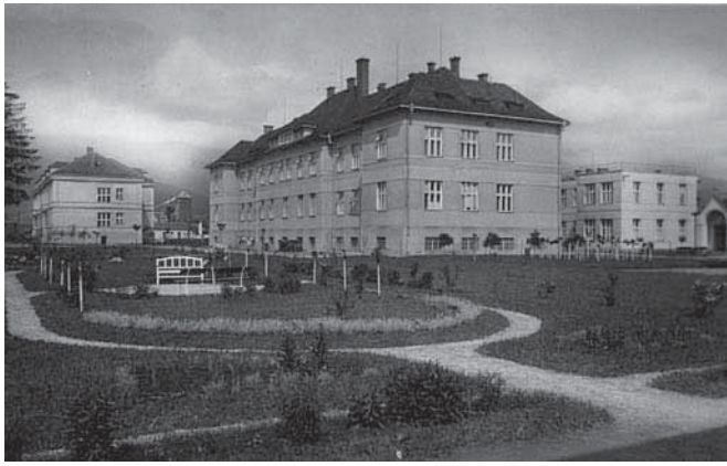
FROM LEFT TO RIGHT: THE INFECTIOUS DISEASES PAVILION (V. HOUDEK), THE SURGICAL PAVILION AND THE OLD SURGICAL (INTERNIST) PAVILION (HLAVAJ – PALKOVIČ – ULIČNÝ) OF THE COUNTY HOSPITAL IN MARTIN
