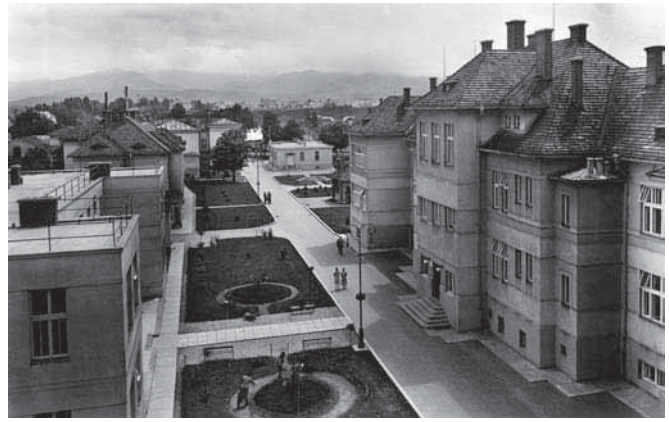
THE OLD SURGICAL PAVILION AND THE NEW SURGICAL PAVILION OF THE COUNTY HOSPITAL IN MARTIN, HLAVAJ – PALKOVIČ – ULIČNÝ, 1928
